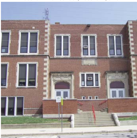
EVERTS MIDDLE SCHOOL, CIRCLEVILLE, OHIO
